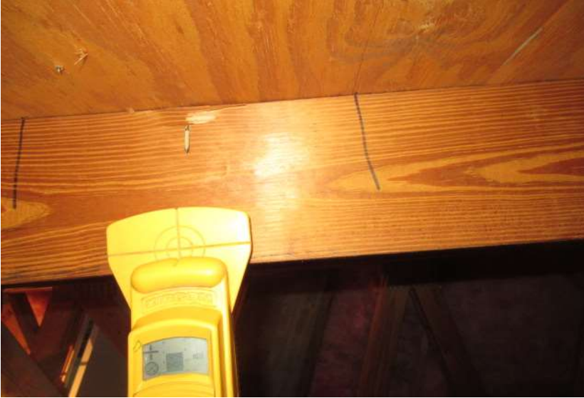
Nail location verified
